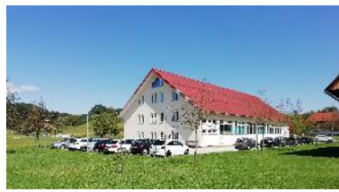
Plant in Vrbeno, Slovenia
